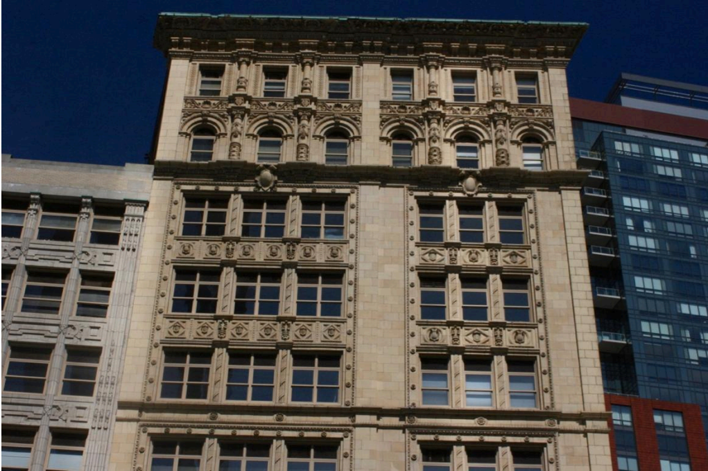
Figure 6. Washington Street façade, floors 6 through 10.
