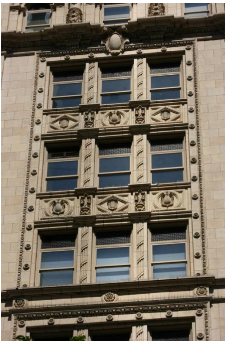
Figure 7. Washington Street façade, detail of floors 6, 7, and 8.
