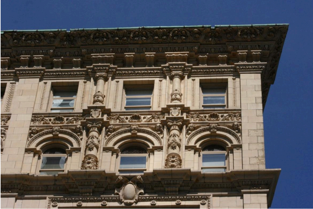
Figure 8. Washington Street elevation, detail of floors 9 and 10.
