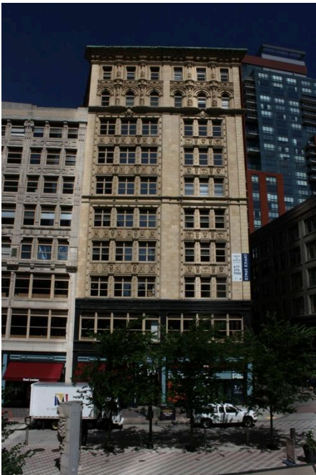
Figure 3. Two-bay Washington Street (east) façade.
