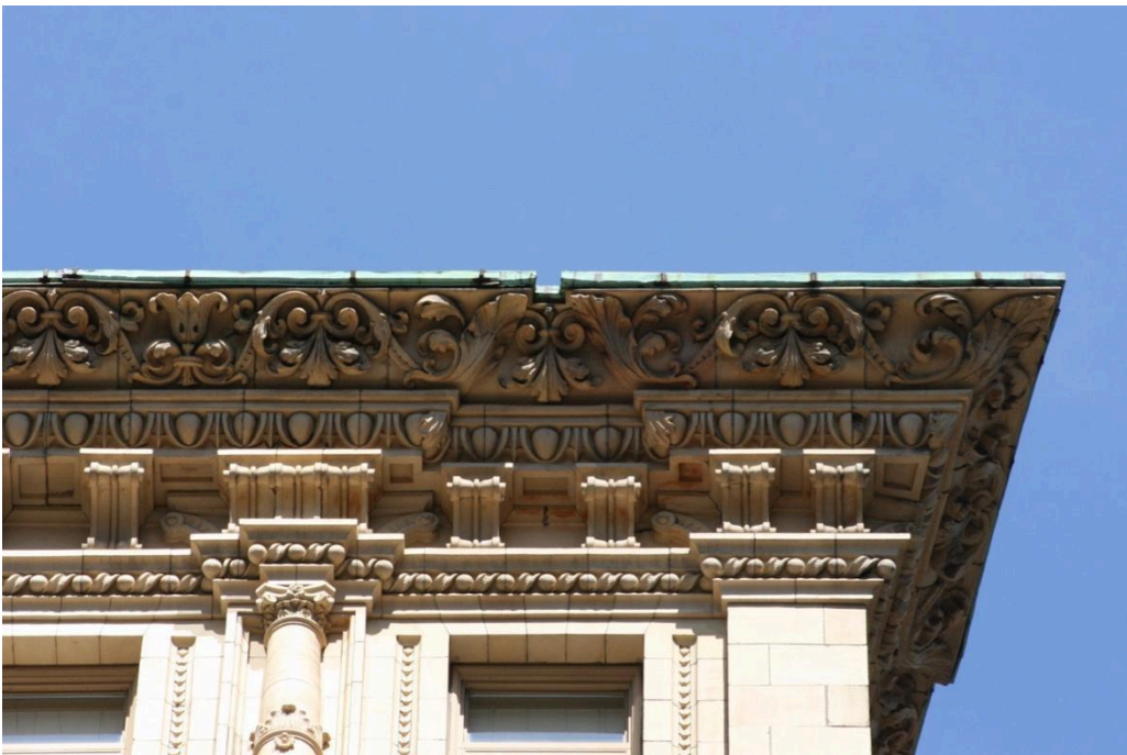
Figure 9. Washington Street elevation; detail of cornice.
