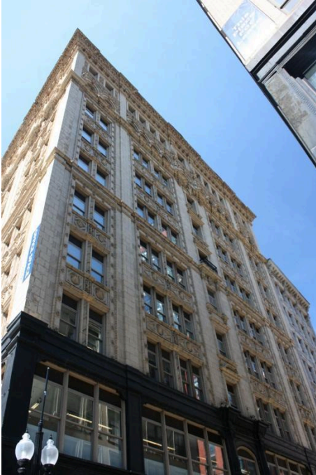
Figure 4. Bromfield Street (north) façade.
