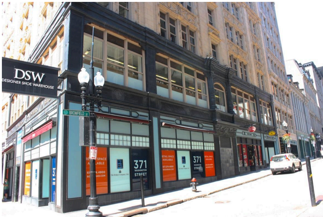
Figure 5. Bromfield Street facade, storefronts.
